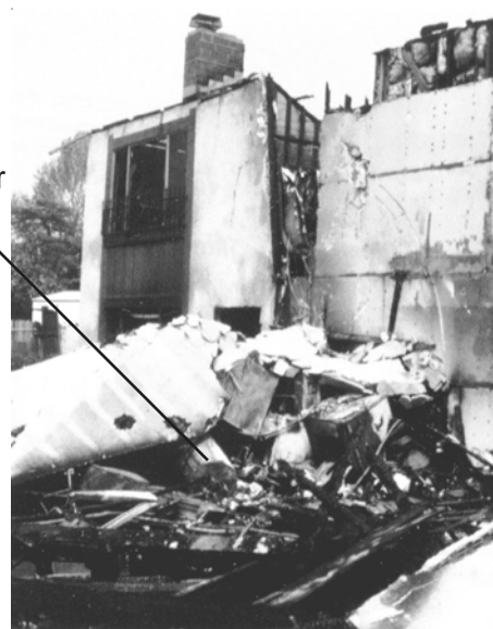
Figure 10 - The unbraced water heater in this home fell during an earthquake; the resulting fire destroyed the home.
